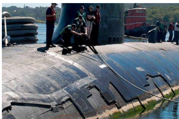
A 2010 photo of the side of the USS Virginia appears to show that the Special Hull Treatment peeled off while the submarine was underway. (U.S. Navy photo)
